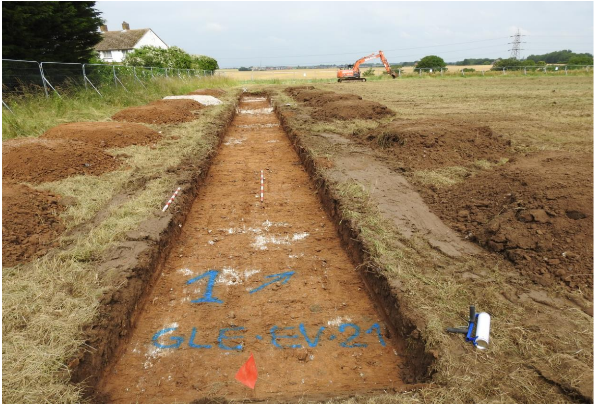
Plate 3: Trench 1 looking north-west with two metre scale.
