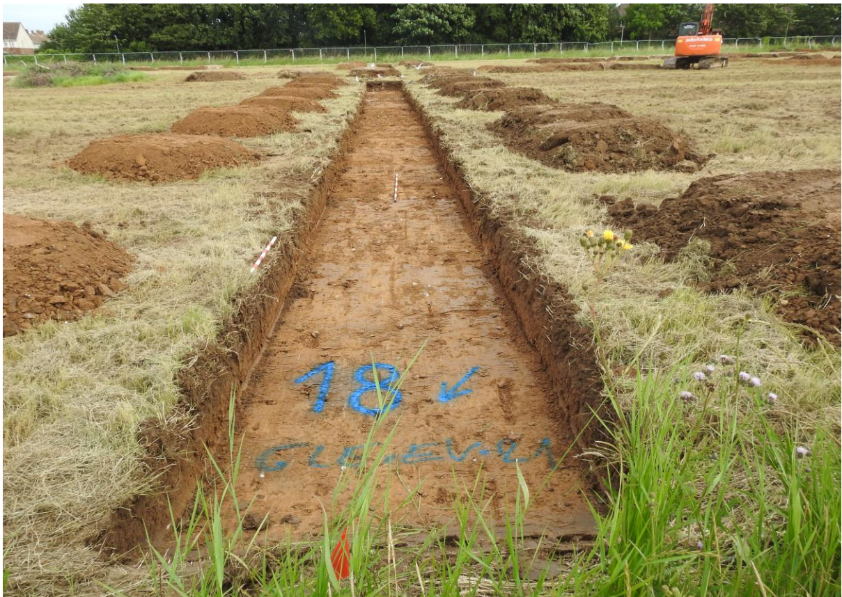
Plate 22: Trench 18 looking south-east with two-metre scale.
